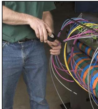
Pull a couple of feet of each cable through the cable sorter.
